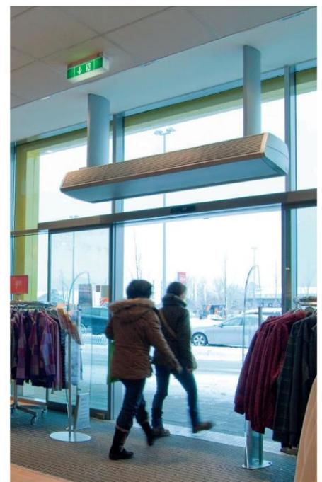
**Figure 2** Air curtain: maintaining comfort conditions with doors open.
